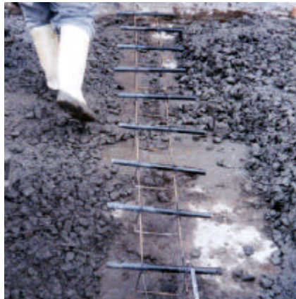
Figura 30. Refuerzo transversal varilla lisa 1" L = 0.33M @ 0.30M.
