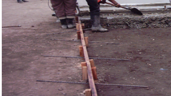
Figura 49. Refuerzo transversal var. lisa 1" L = 0.45 m @ 0.3 m
