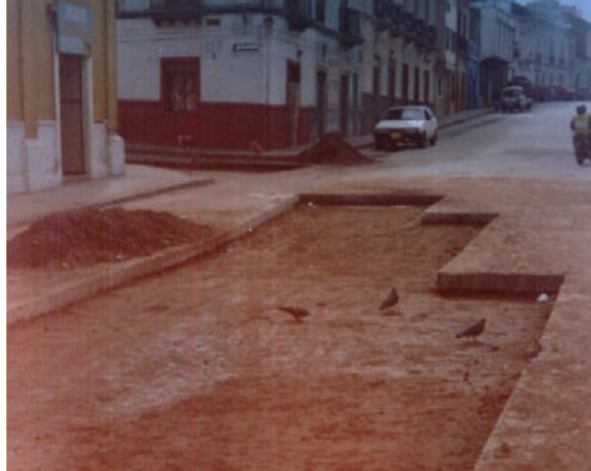
Figura 65. Base granular, E = 0.20 m
