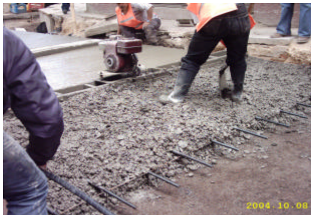
Figura 49. Refuerzo transversal var. lisa 1" L = 0.45 m @ 0.3 m
