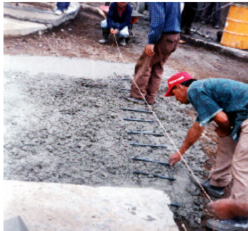
Figura 67. Refuerzo transversal varilla lisa 1" L = 0.45 m @ 0.30 m.
