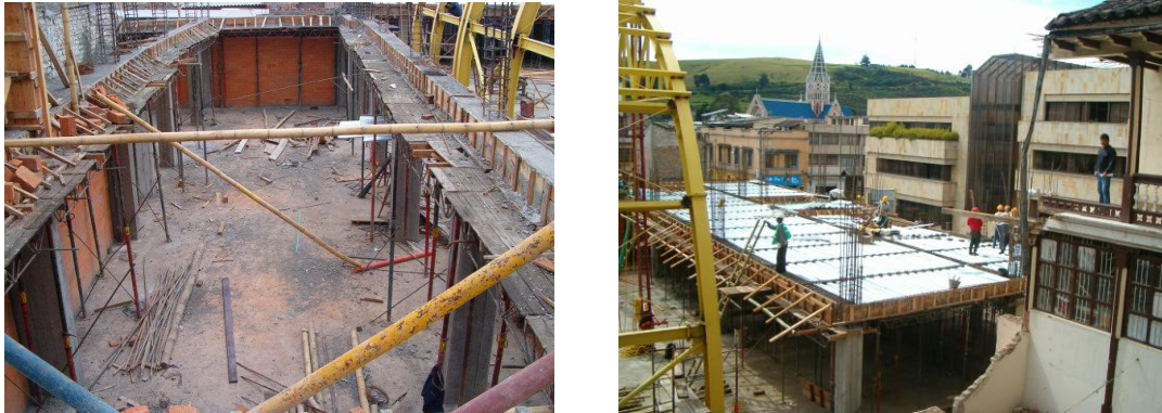
Figura 64. Vigas aéreas n+3.50 – mezanine.
