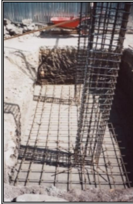
**Figura 132. *Zapata Fundida***
