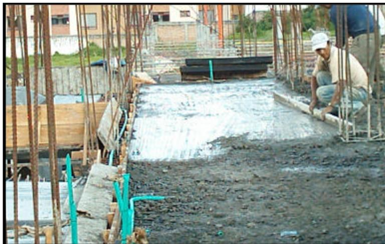
Figura 109 . VISTA GENERAL LOSA FUNDIDA E = 0.40 MT
