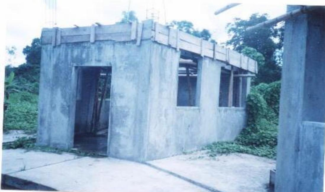
**Figura 54. Encofrado Vigas Aéreas (0.30 x 0.30) m**
