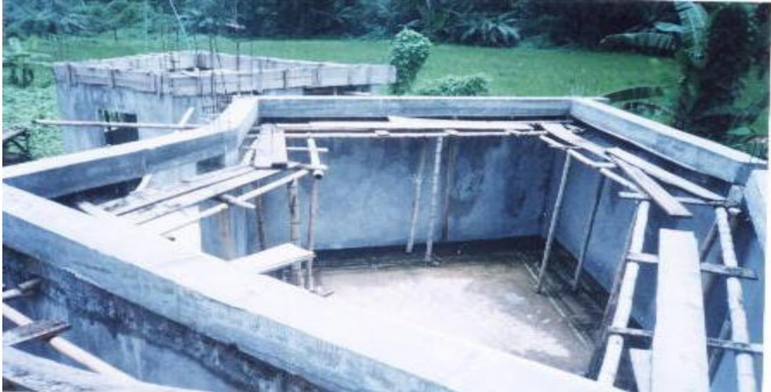
**Figura 56. Vigas Aéreas Fundidas (0.30 X 0.30) m**
