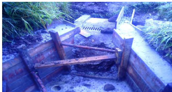
Figura 1. Formaleteo muros laterales bocatoma la Merced.
