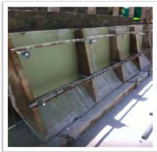
Figura 88: New jersey y baranda peatonal
