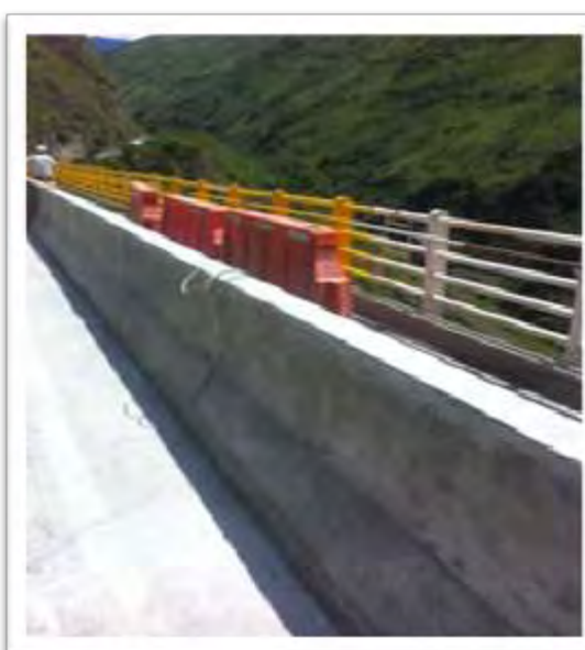
Figura 89: New jersey y baranda peatonal
